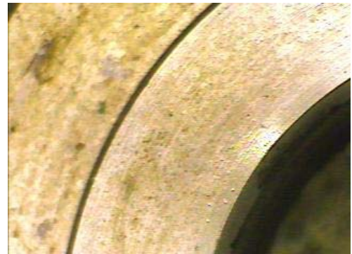
Pitting on Flange Face
